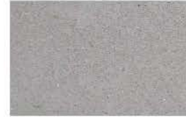
CONC-1 / CONC-2 SEALED CONCRETE
